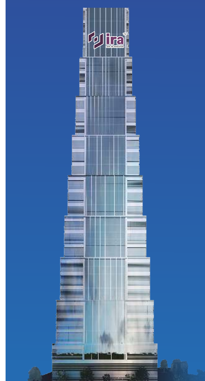
GATEWAY TOWERS, PUPPALAGUDA
